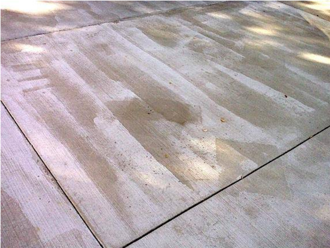
Improper sealer application with a roller
