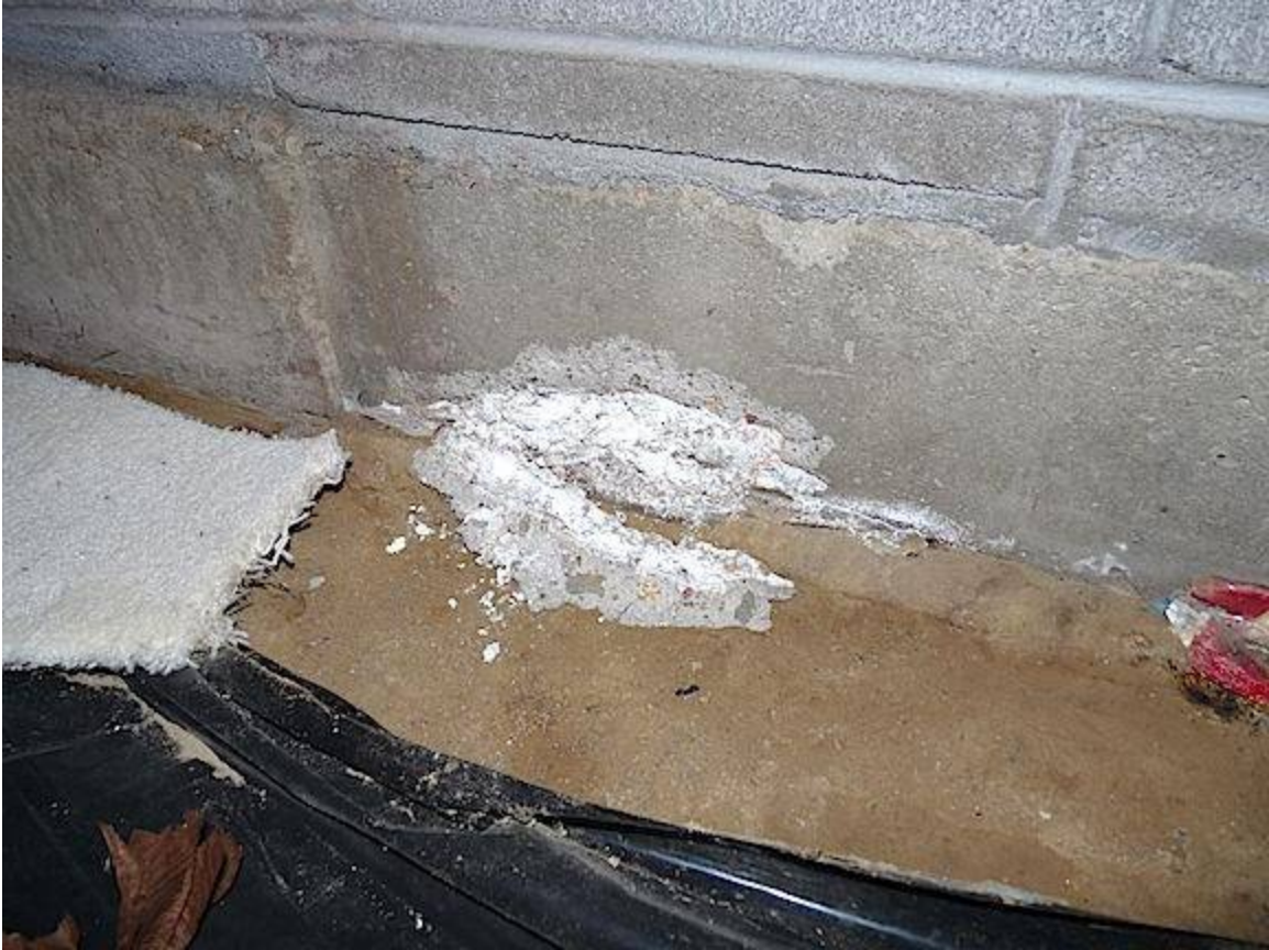
Flaking at a crawlspace footing
