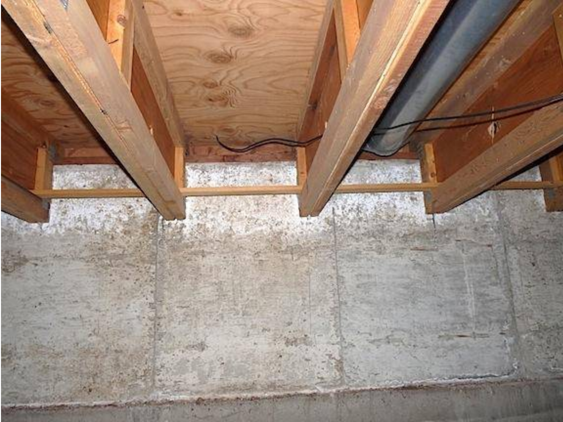
Efflorescence from neutral grade
