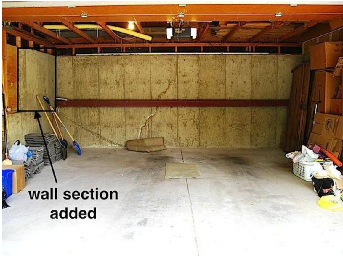
A section of the concrete foundation wall at the left was extended (the black rectangle).
