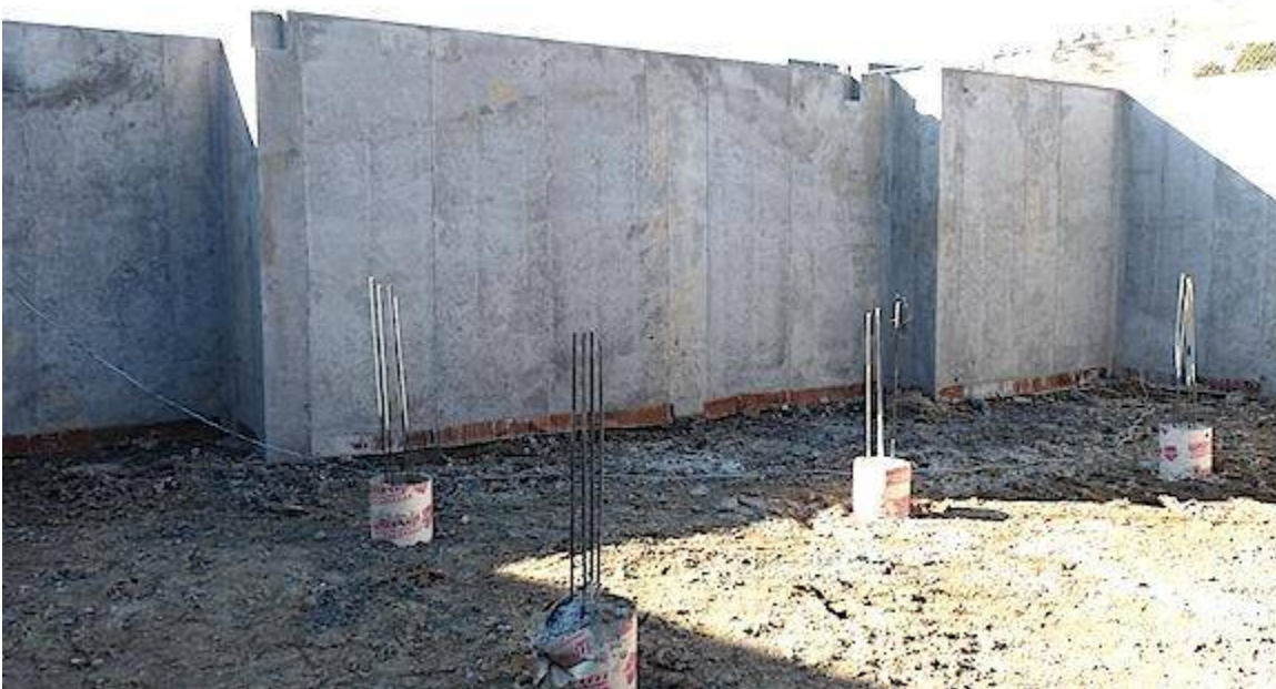
Void forms after the walls have been poured
