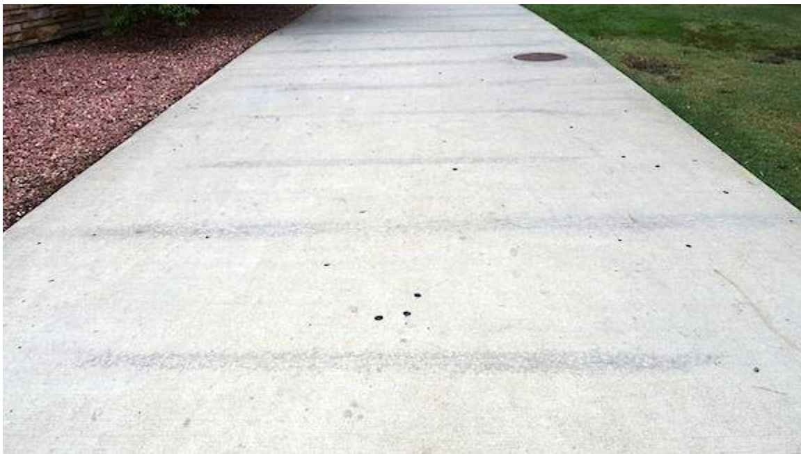
Repeating pattern of cracks where rebar cross-members connect longitudinal rebar
