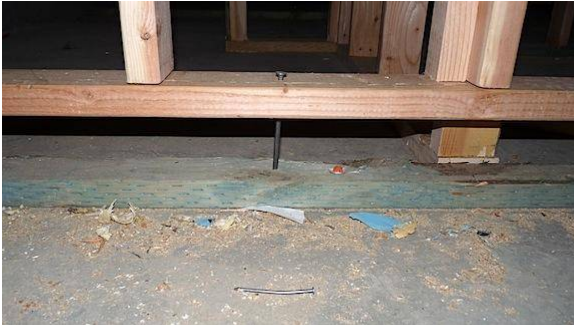
A doubled bottom plate connected to a wall with a single bottom plate
