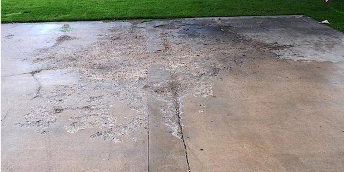
Smaller patches of damage have expanded to form a large area of damage.
