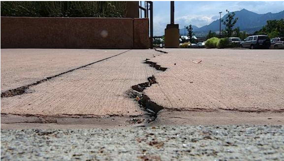
Vertical displacement occurred as the lower end of the walkway settled.
