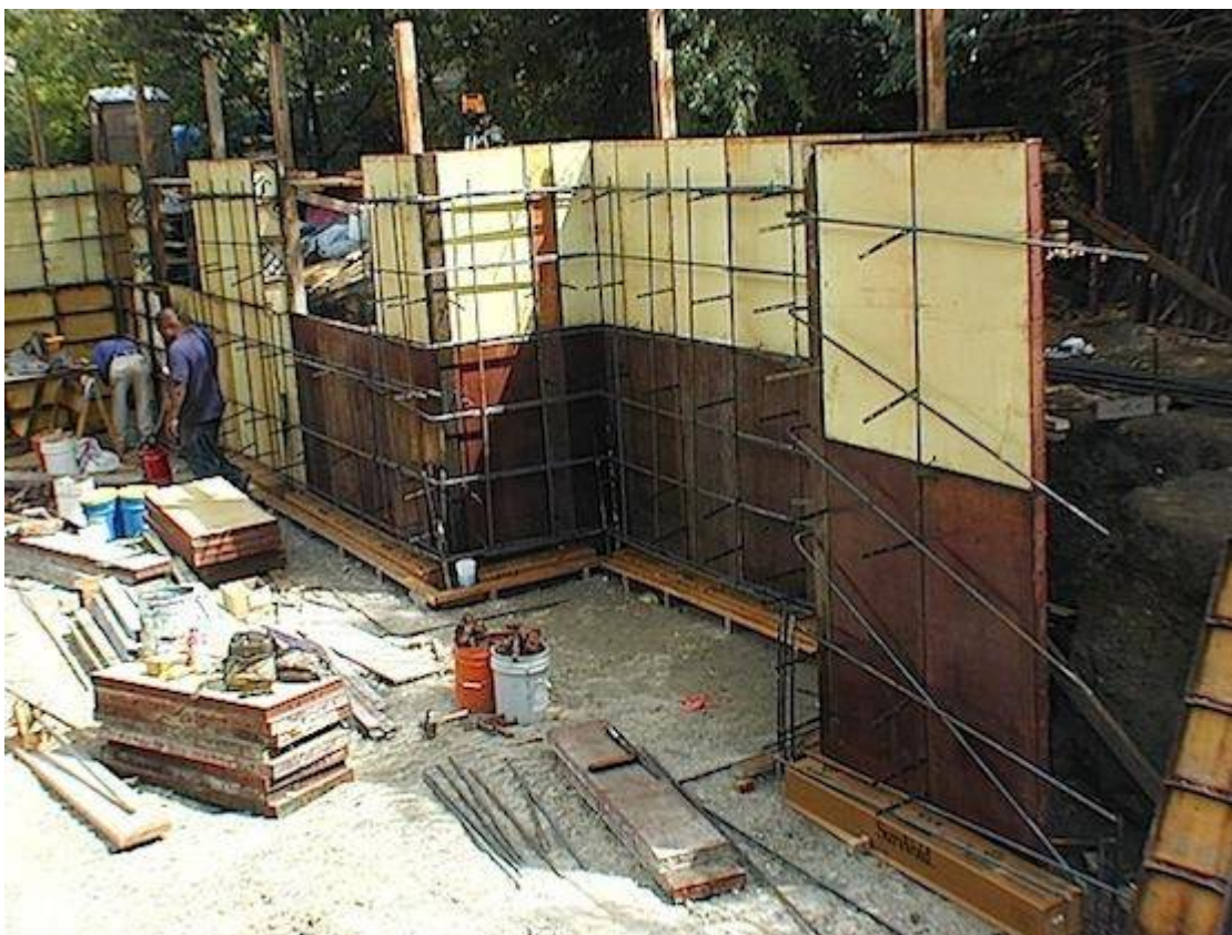
This drilled-pier foundation will be placed on void forms and piers that are resting on bedrock.
