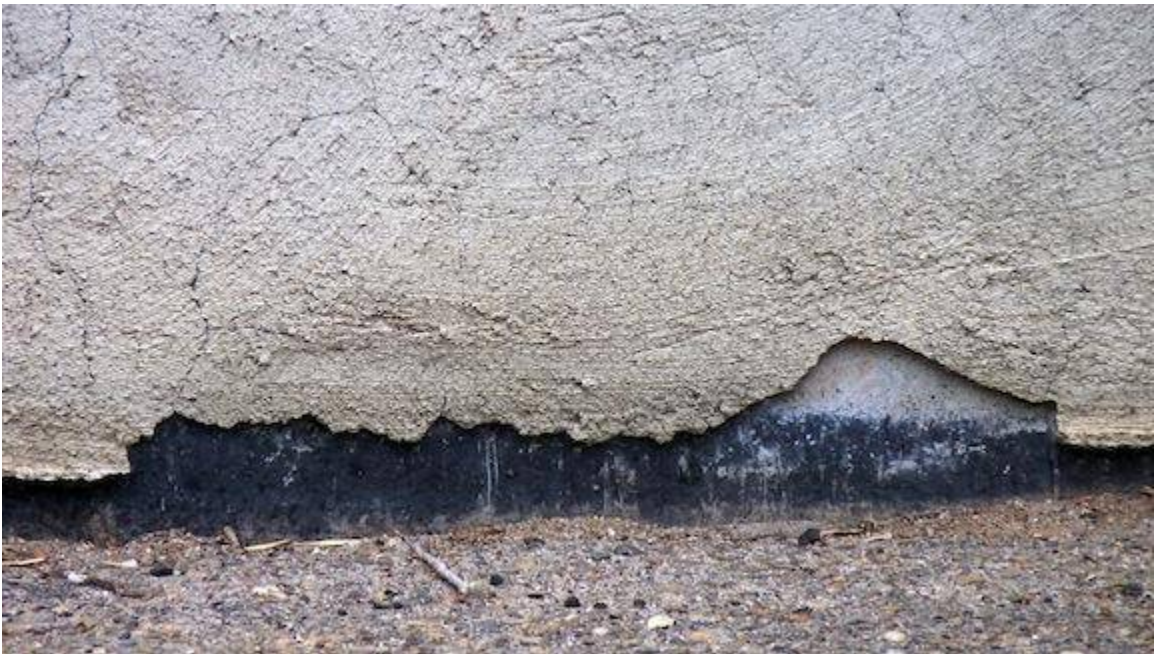
The photo above shows a close-up of the parge coat. The parge coat bond has failed and it has begun to delaminate from the underlying wall.
