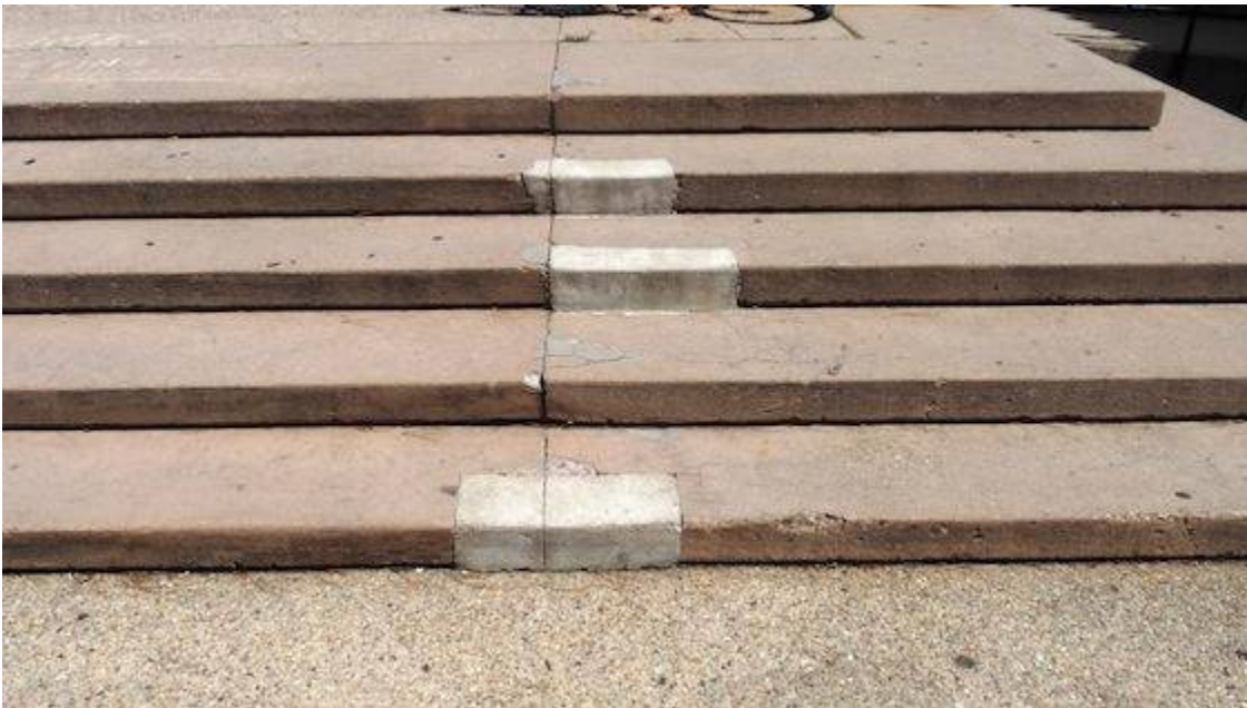
Poor-quality repairs may result in the re-appearance of corrosion.
