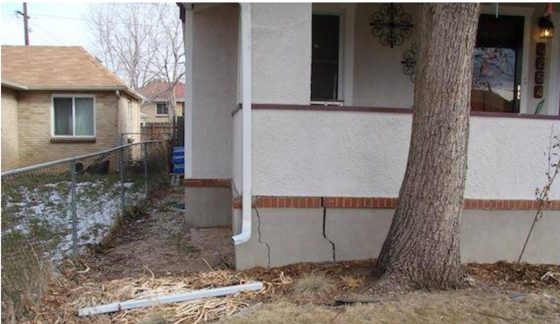
An example of differential settling
