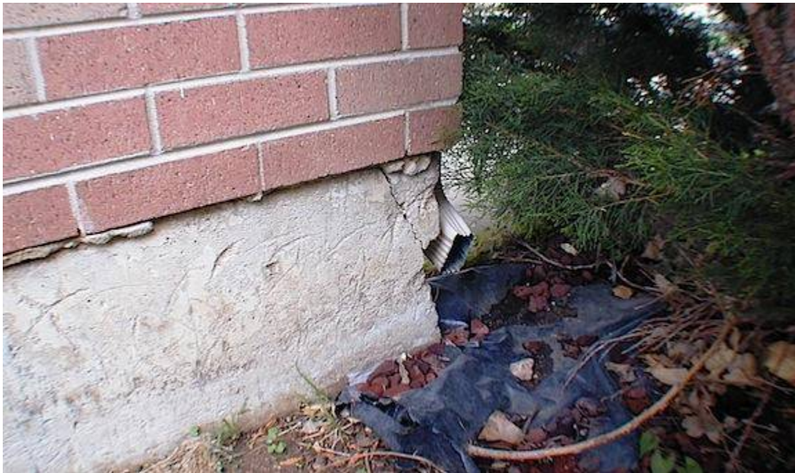
Outside corners are also high-stress points.
