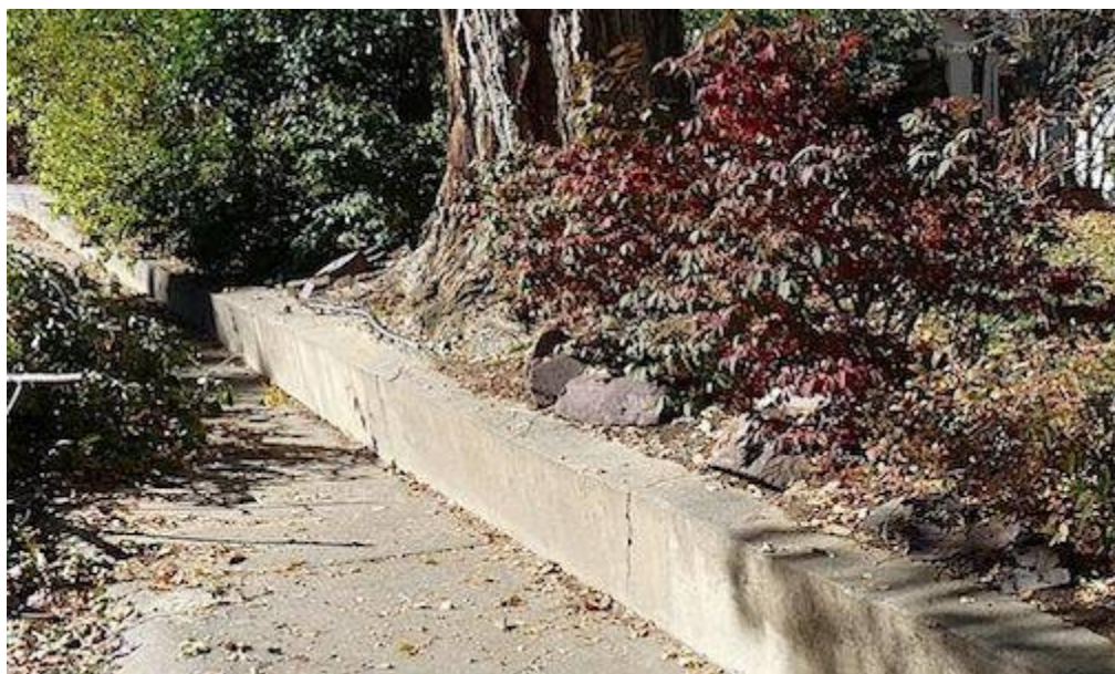
Creep with cracking
