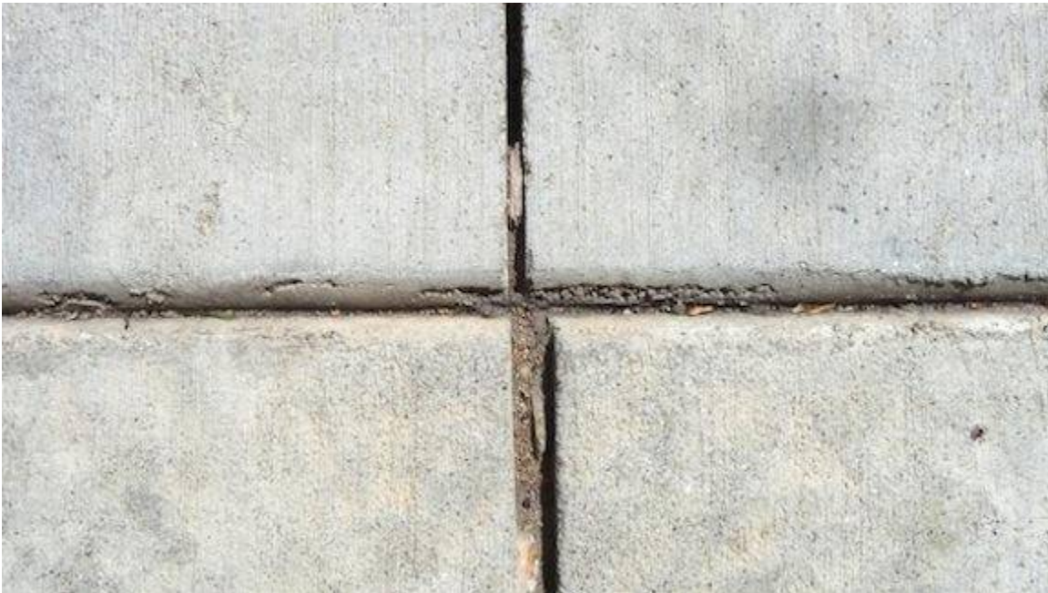
The vertical joint is a sawn joint and the horizontal joint is tooled.
