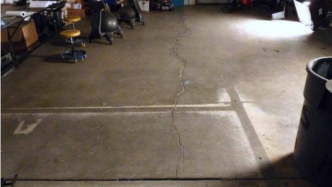
Notice the lack of control joints in this shrinkage crack.
