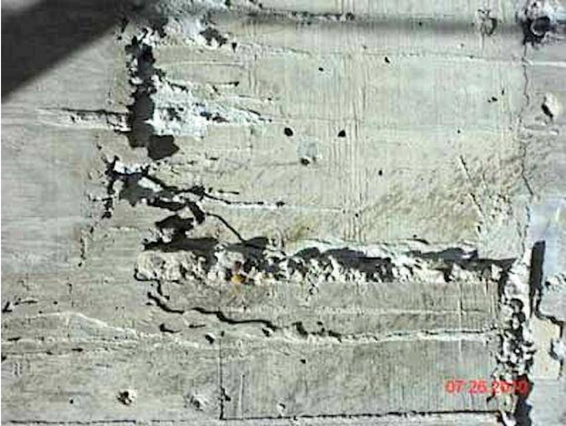
A cold joint in concrete
