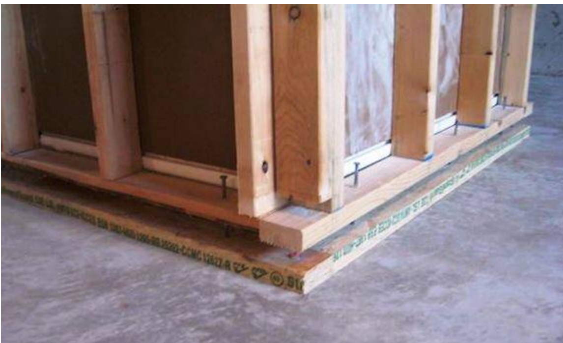
The doubled bottom plate accommodates heaving.
