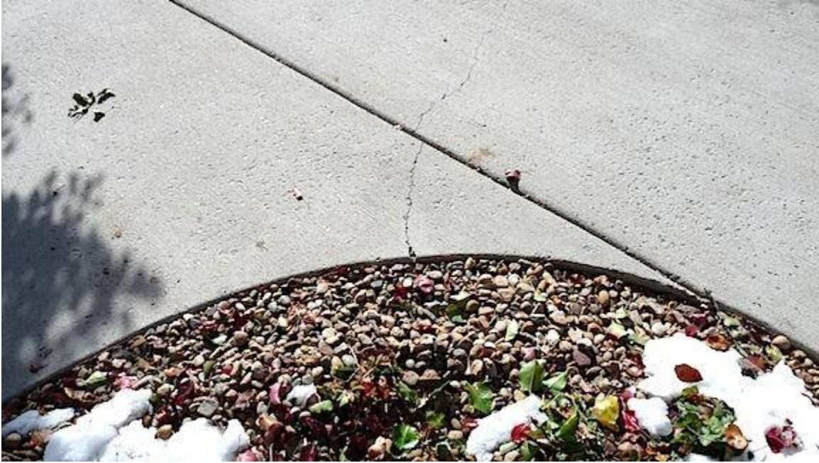
Re-entrant cracking at the apex of a radiused re-entrant corner
