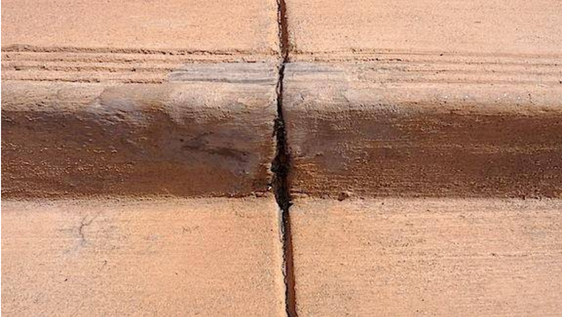
Repairs are common at control joints in stairs at well-maintained properties.
