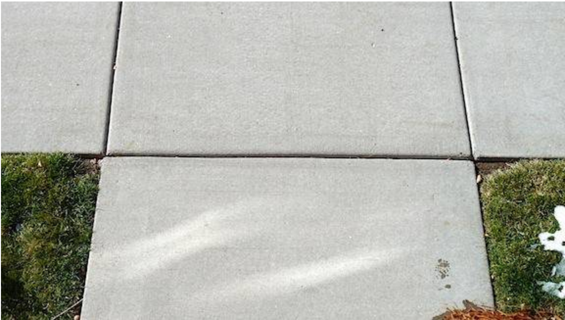
A re-entrant corner with properly placed control joints
