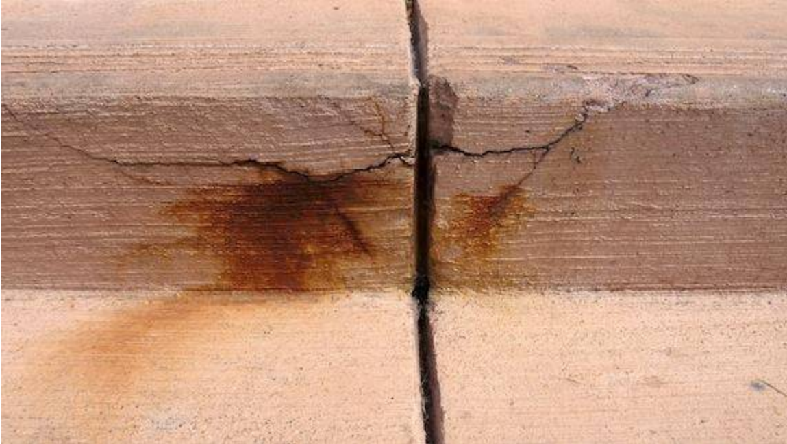
Concrete cover will be thinner at control joints.
