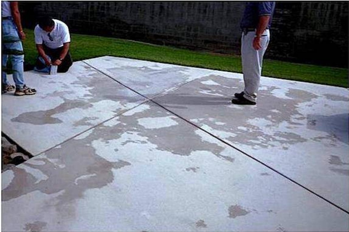
Poor sub-base preparation
