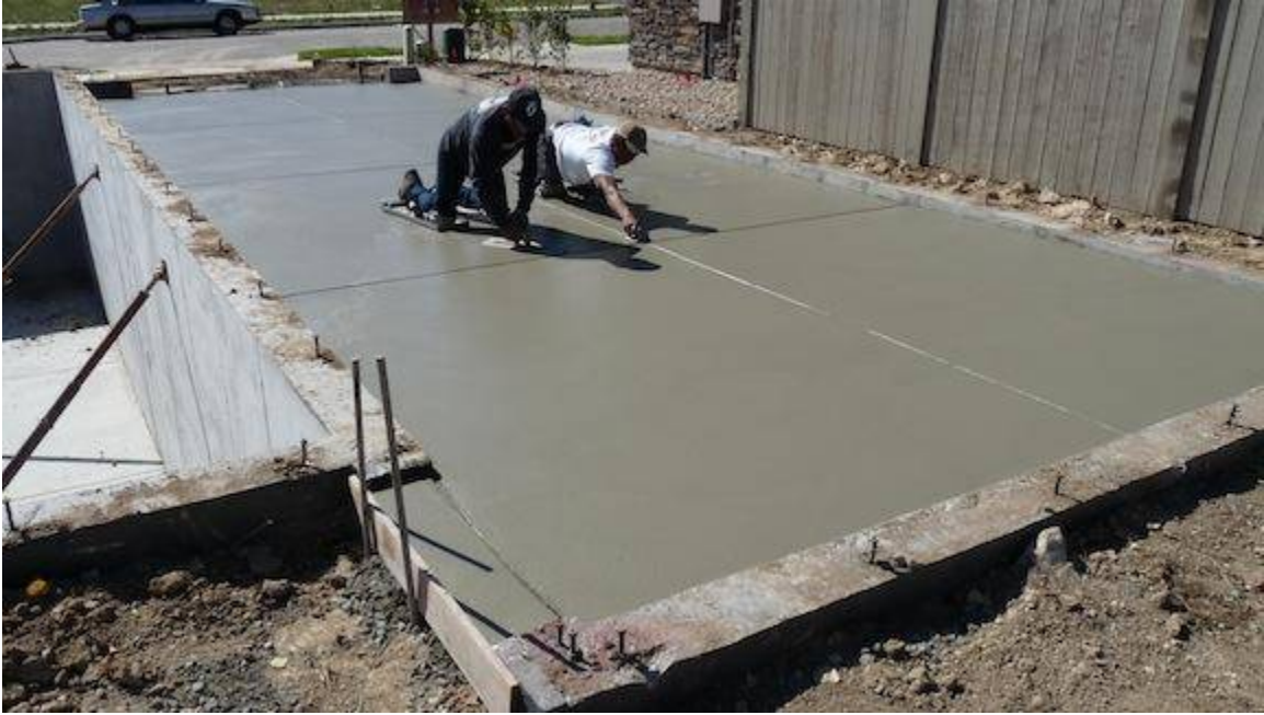
The new floor, which will expand, is contained by the foundation wall.
