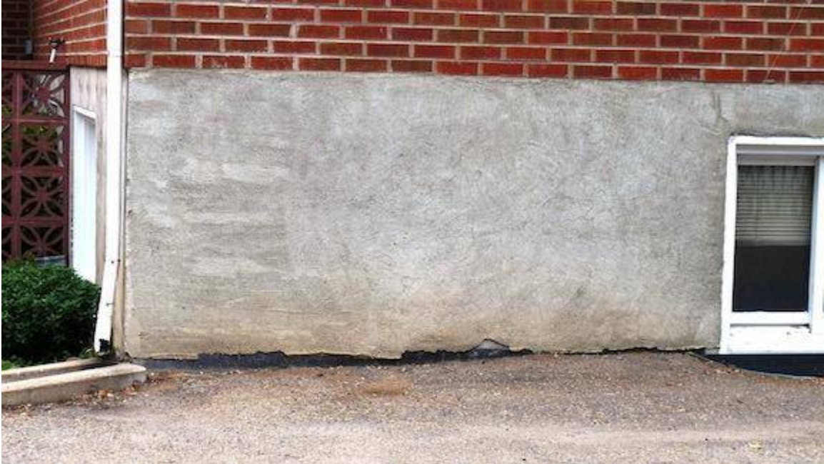
A parge coat showing widespread pattern cracking from excessive water in the mix or excessively fast drying, or both
