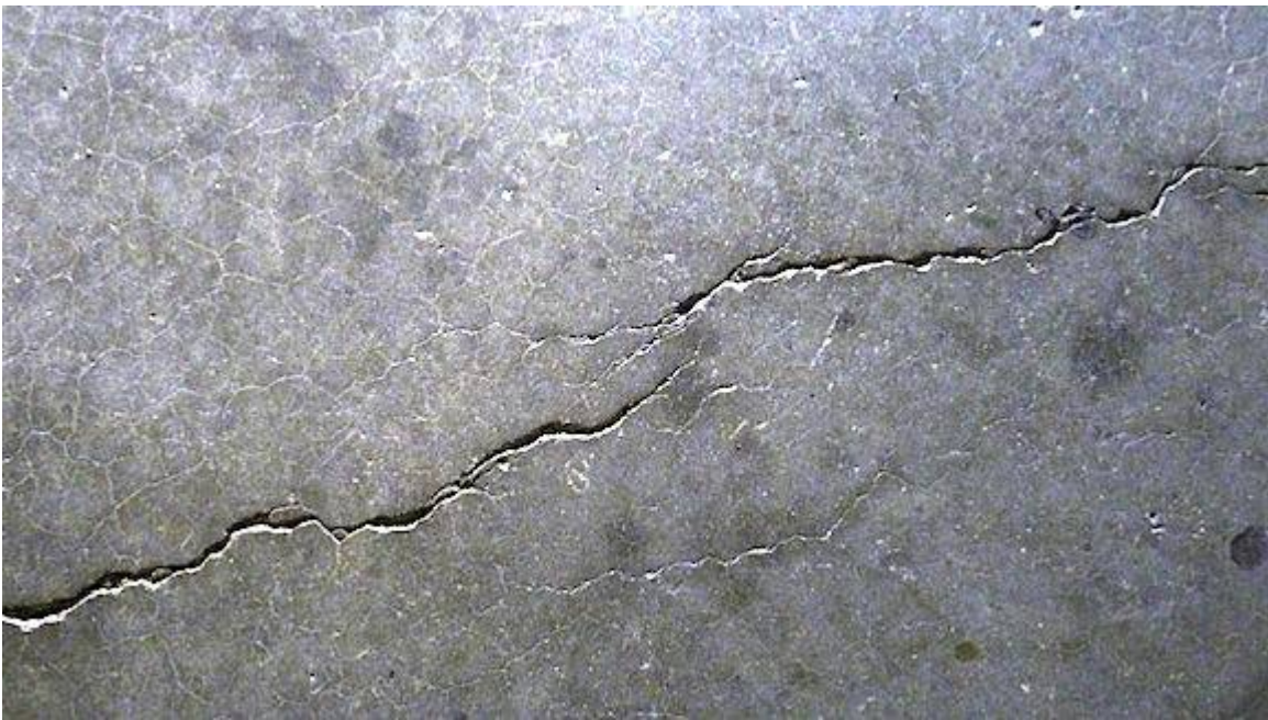
A typical interruption in a shrinkage crack
