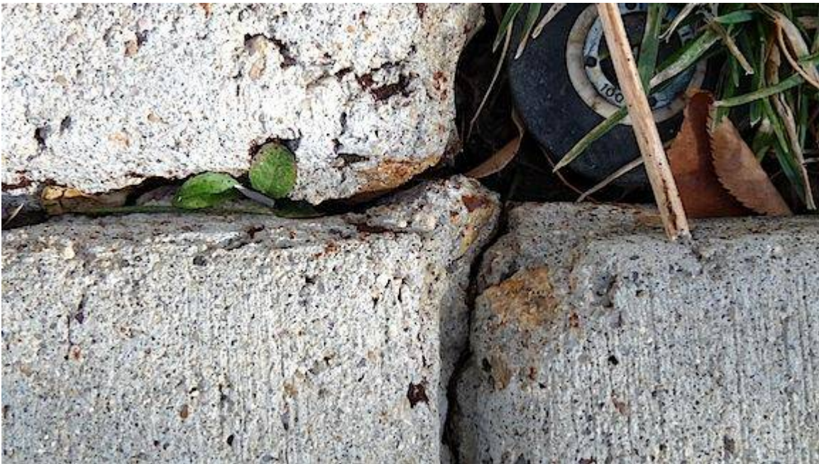
This close-up of the corner shows cracking taking place in the control joints, as it should.
