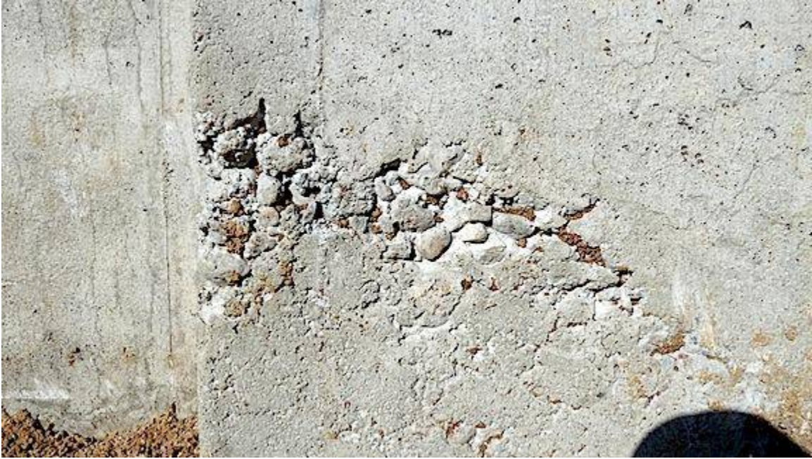
Honeycombing due to poor consolidation
