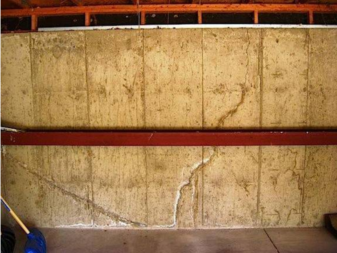
A steel I-beam acts as a strongback. (The top flange of the beam is facing the camera).
