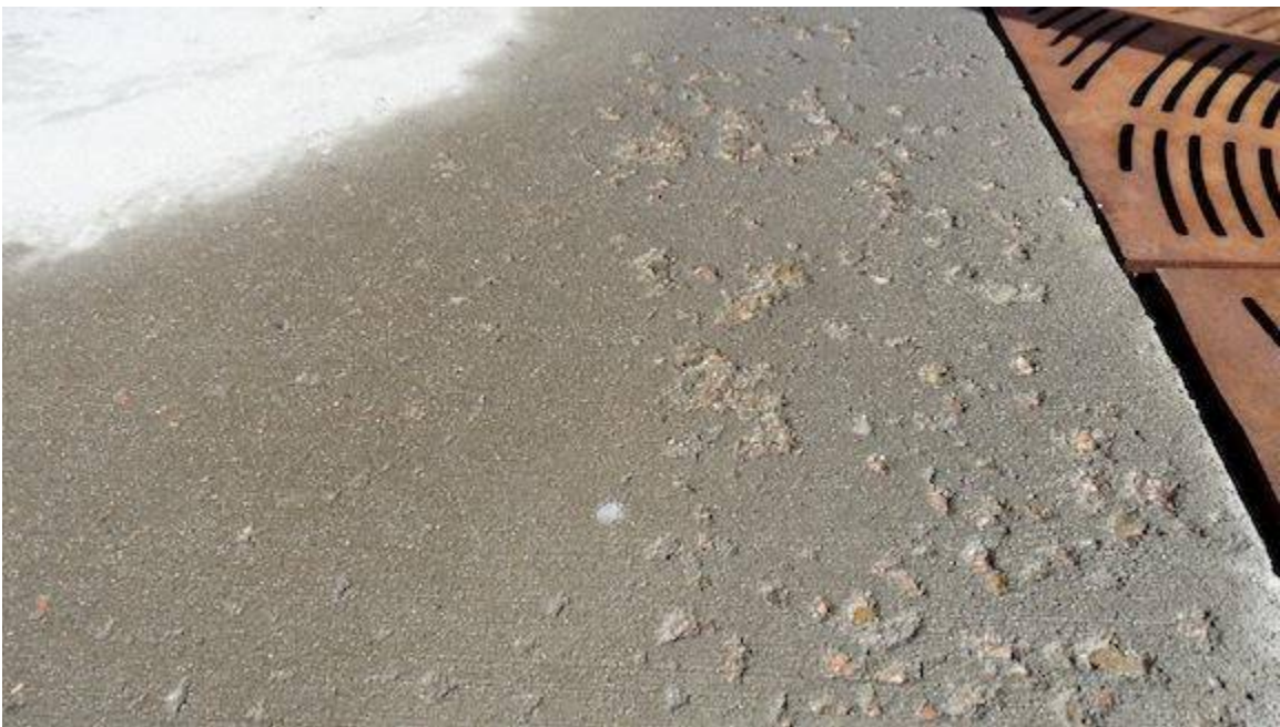
The lack of ruptured aggregate indicates that this damage was most likely caused by reactive aggregate.
