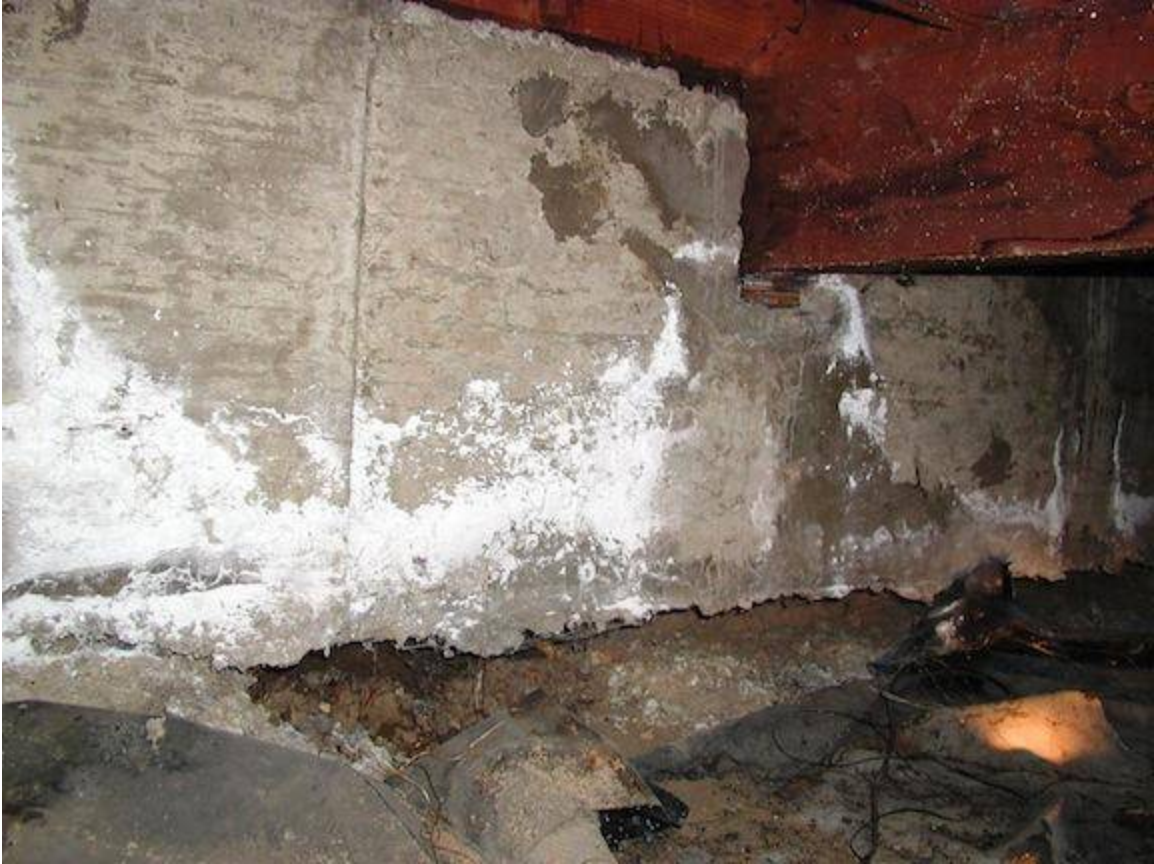
Severe efflorescence from downspout discharge
