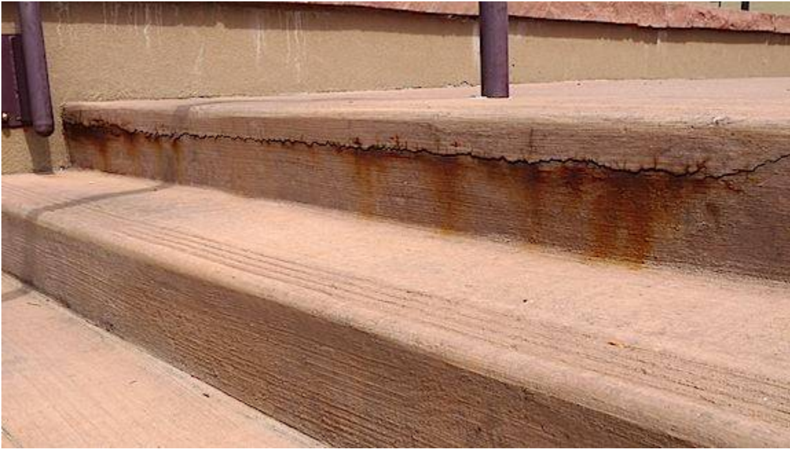
Corrosion typical of inadequate cover
