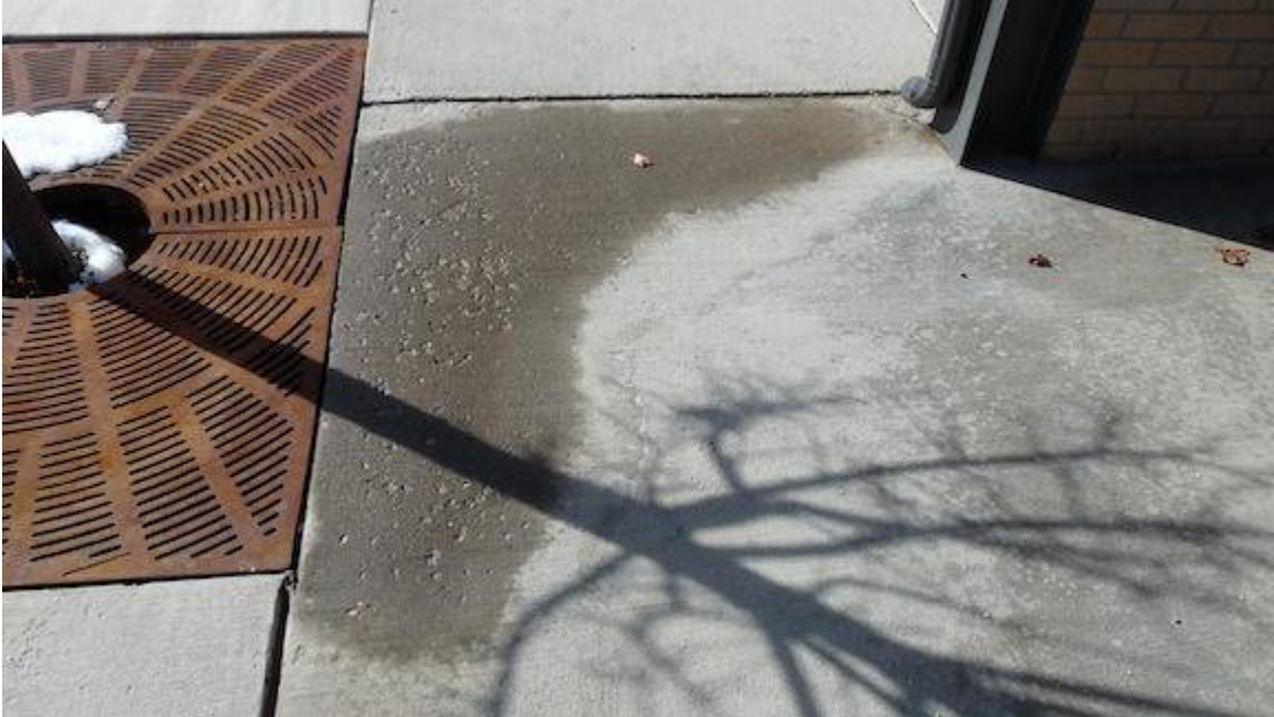
The location of damage reflects the amount of moisture exposure.
