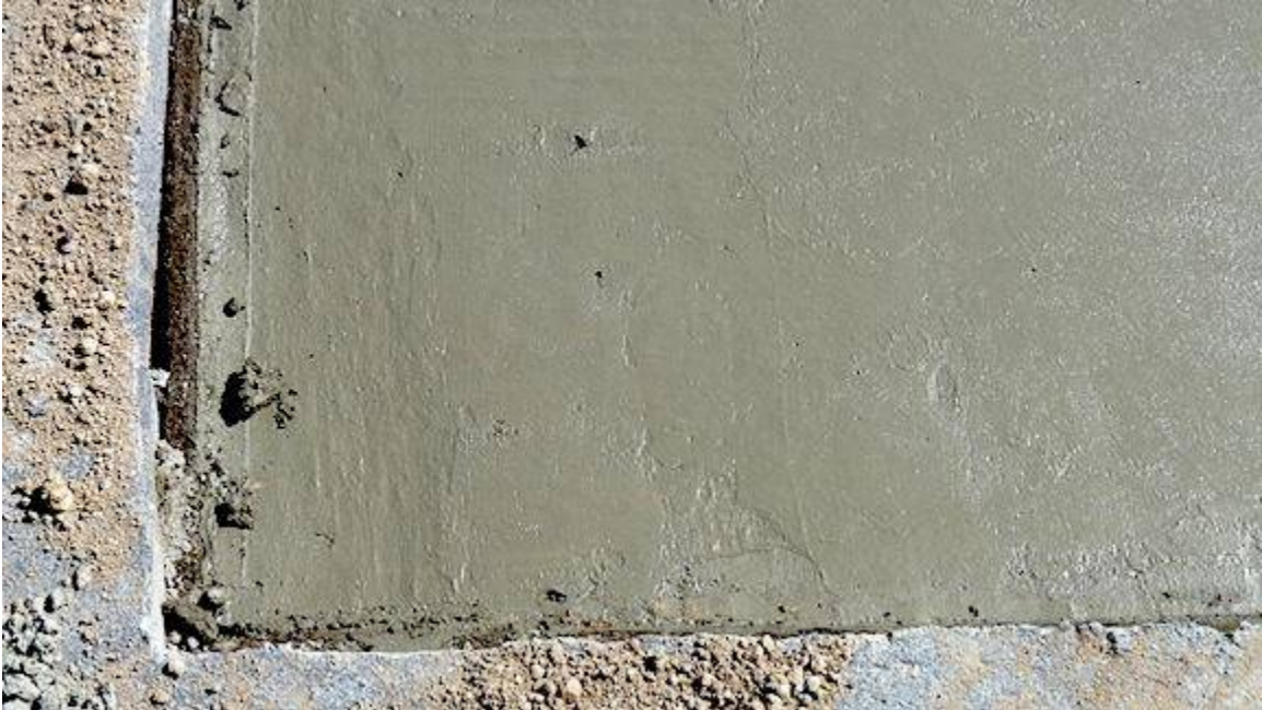
Fibrous isolation-joint material allows the slab to expand without damaging the foundation wall.
