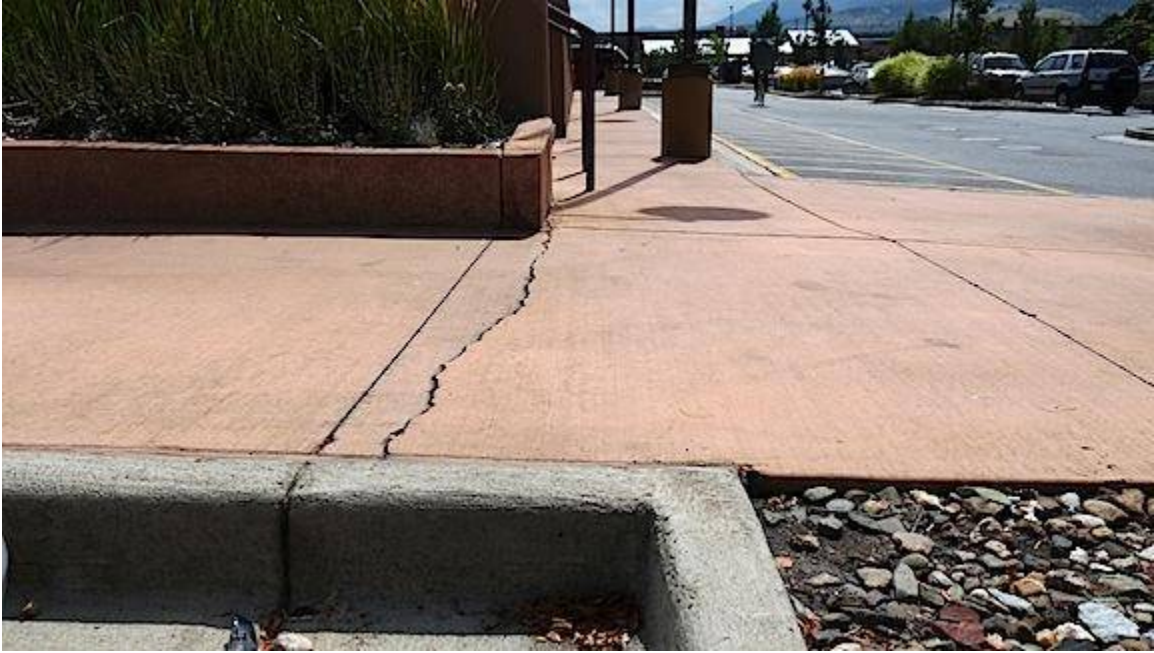
Settling caused by inadequate compaction
