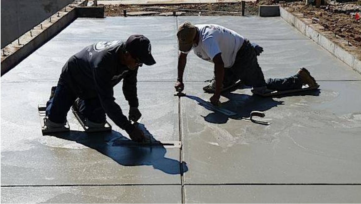
The workman on the right is finish-troweling a tooled control joint.
