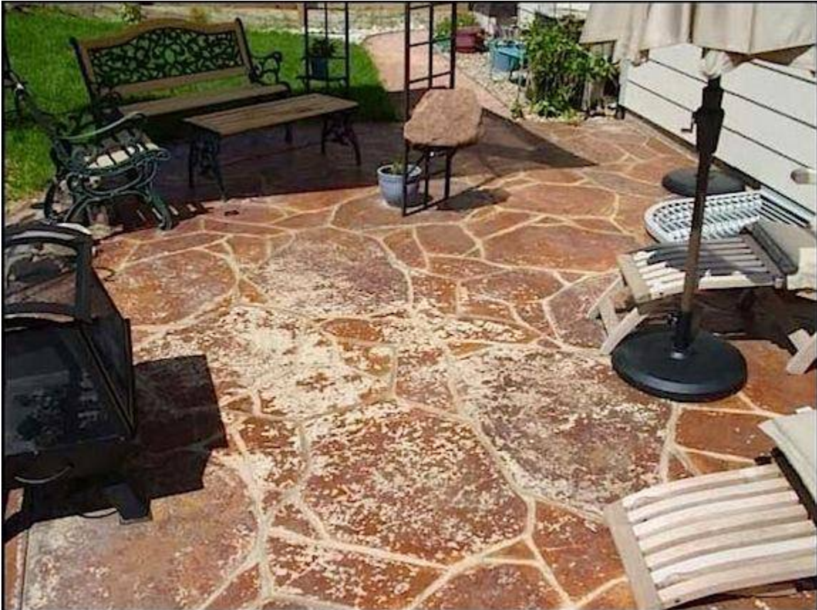
Poor sub-base preparation
