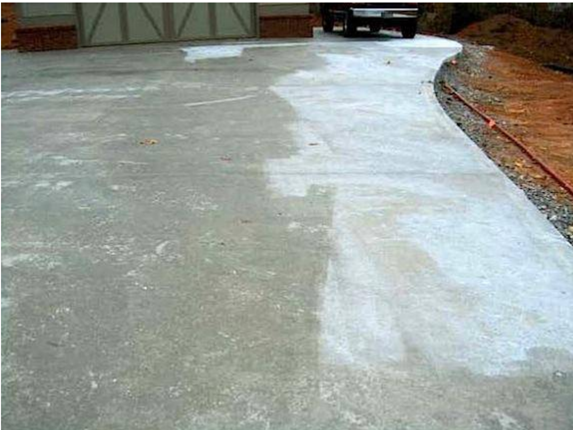
Sealer applied over an excessively wet surface
