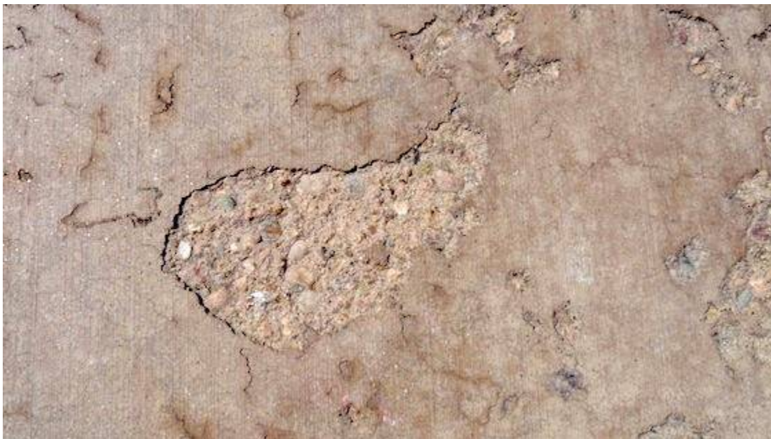
Small patches of flaking
